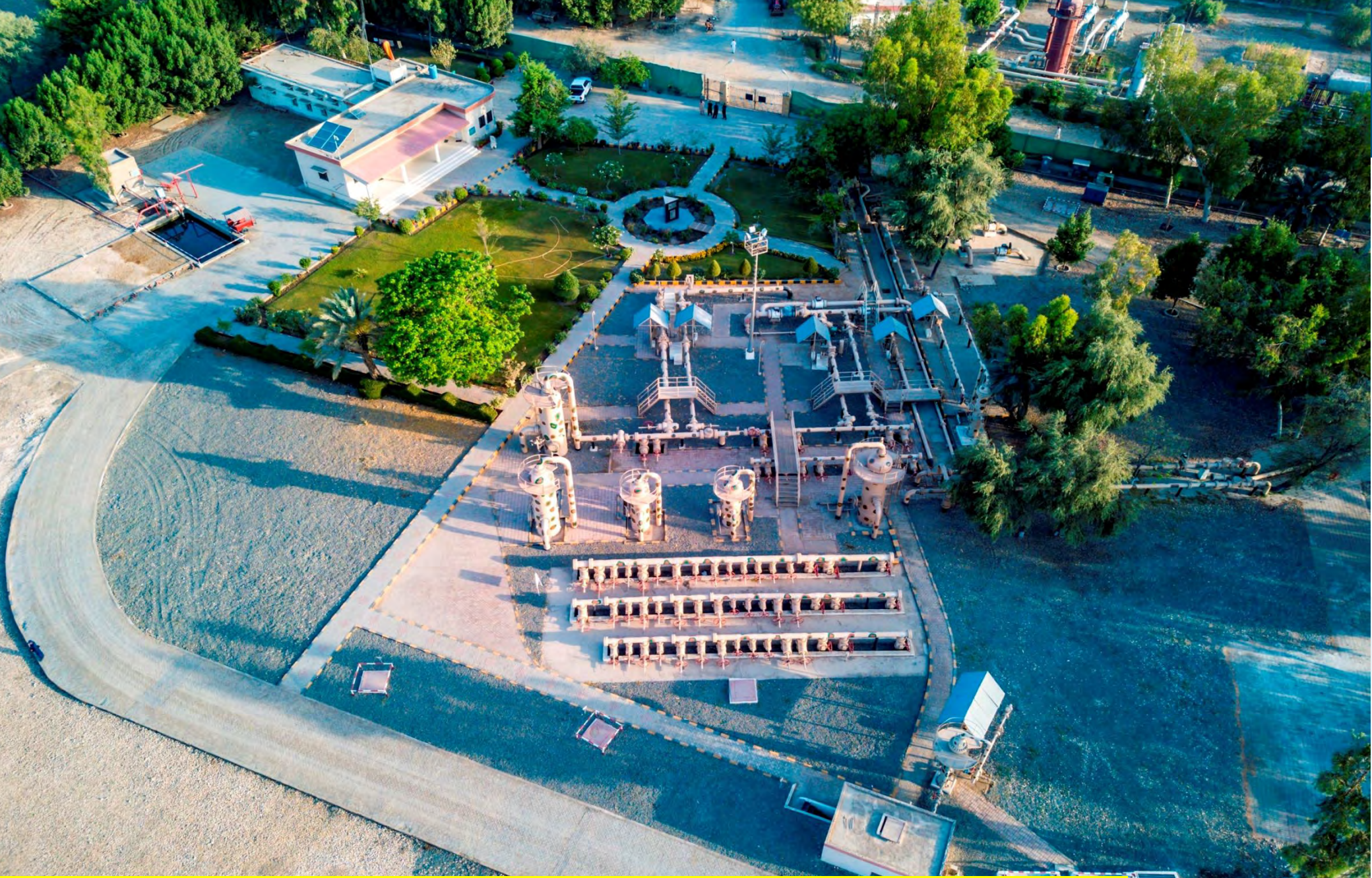
Aerial View of Central Manifold- Mari Gas Field
