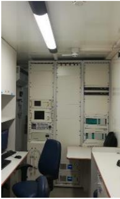
Mud Logging Unit
